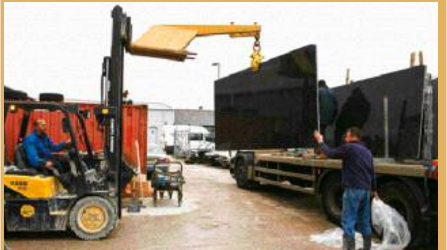
Granite slabs are off-loaded and stacked in the yard. Under-cover storage will soon be increased at the Newton Abbot base so that more marble stocks can be held
