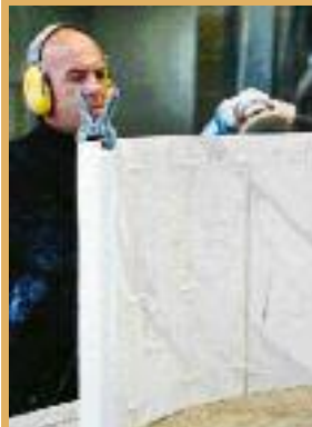
Precision sections of Calacatta Oro marble, sourced from Italy, are glued together to make a curved bath panel for a high-spec bathroom
